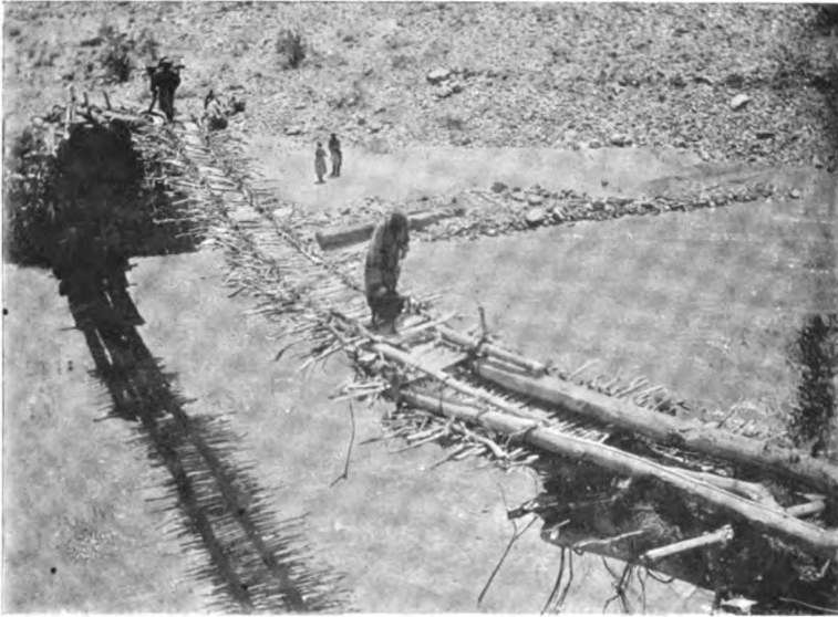
BRIDGE OVER THE BARTANG
